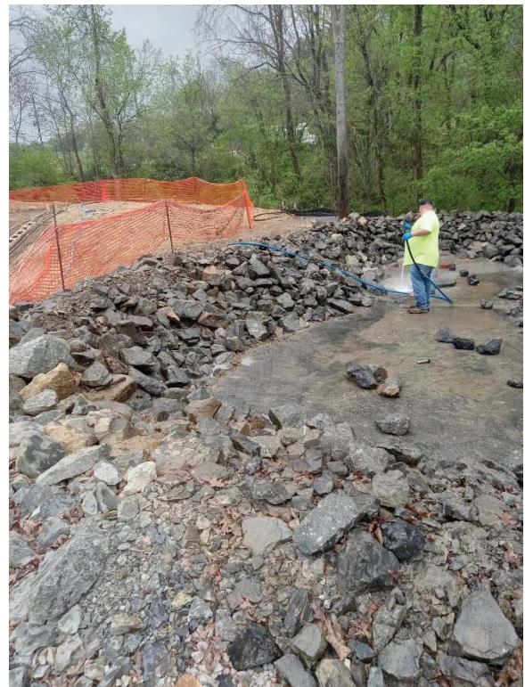
MH 1750 – Hydro-cleaning containment berm
