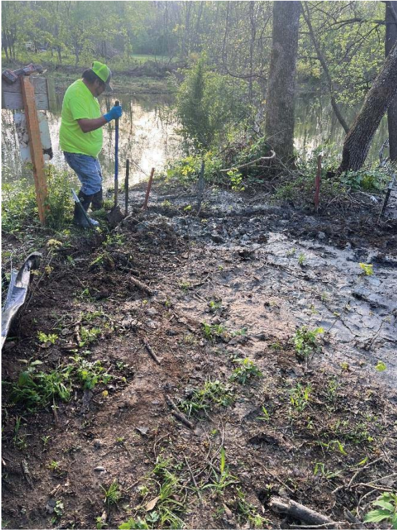
MH 1748 – Removing silt fence
