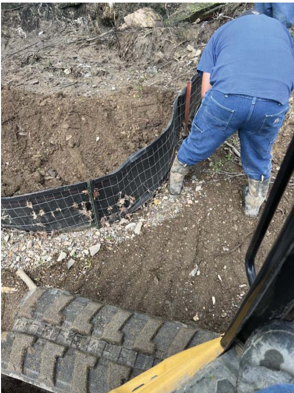
MH 1748 – Installing new silt fence
