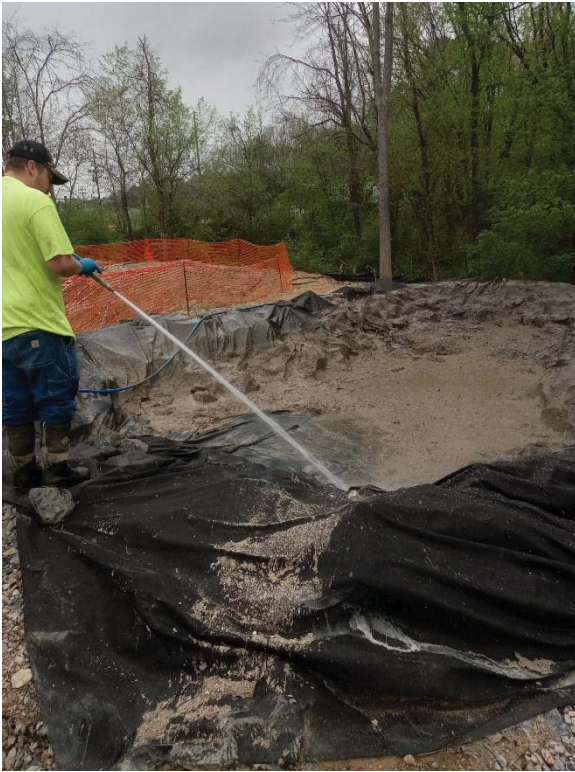
MH 1750 – Hydro-cleaning containment berm
