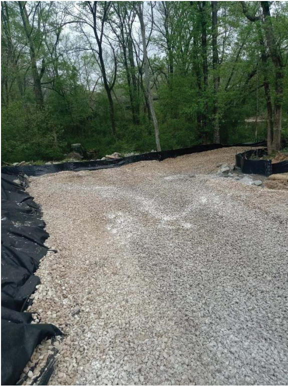
MH 1750 – Access cleanup
