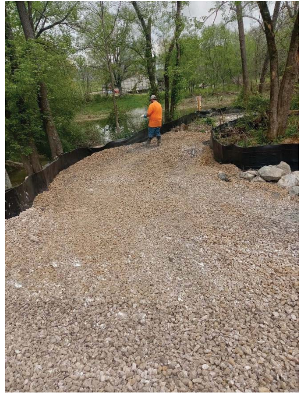
MH 1750 – Access road after cleanup
