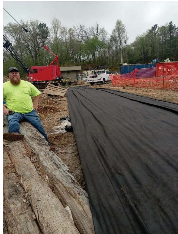
MH 1750 – Installing new liner in berm area
