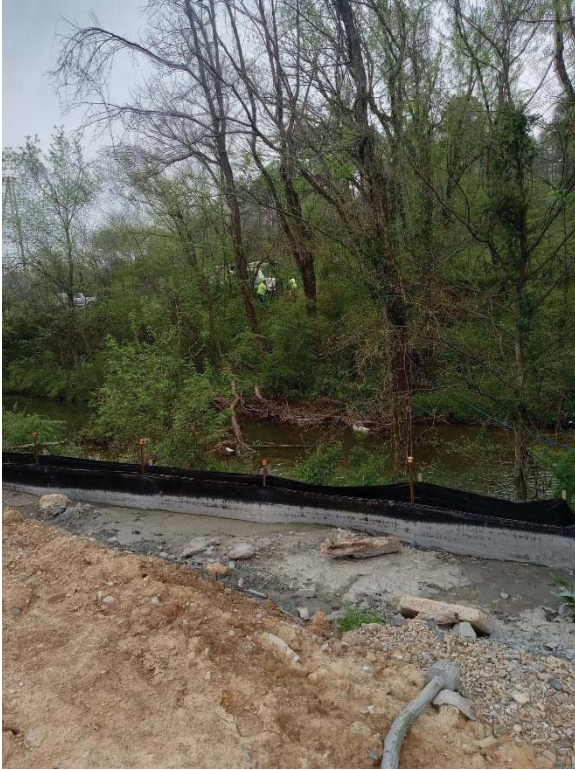
MH 1750 – Silt fence between creek and berm
