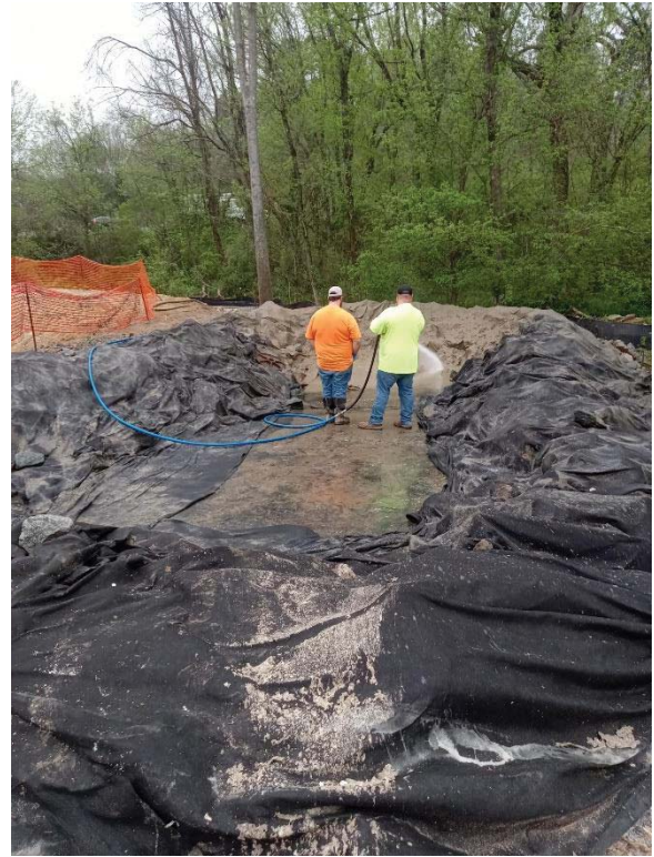
MH 1750 – Hydro-cleaning containment berm
