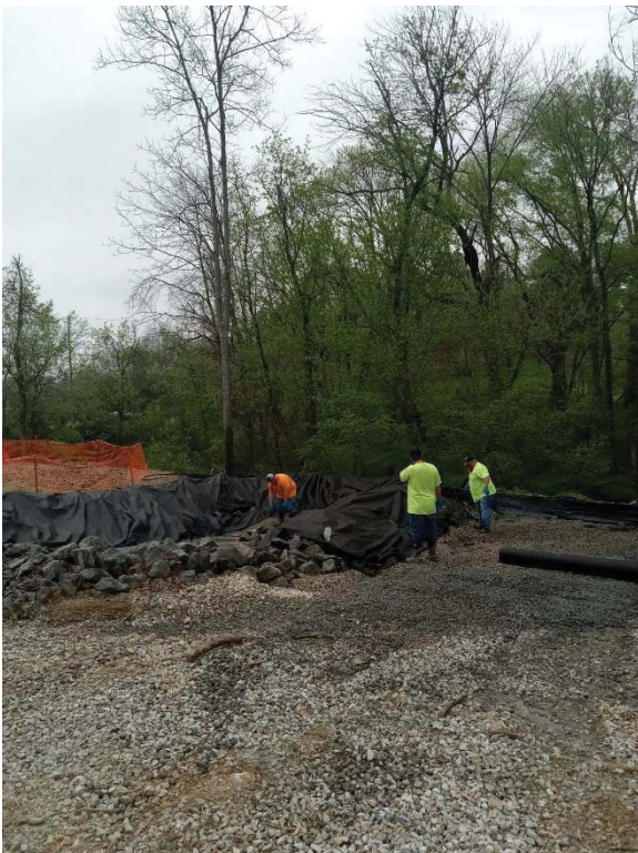
MH 1750 – Installing new liner in containment berm
