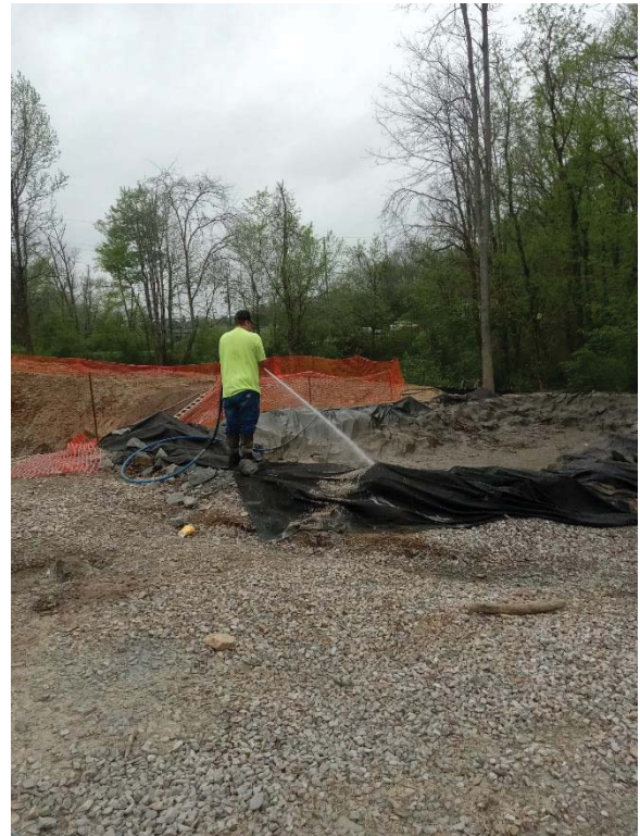
MH 1750 – Washing down inside berm
