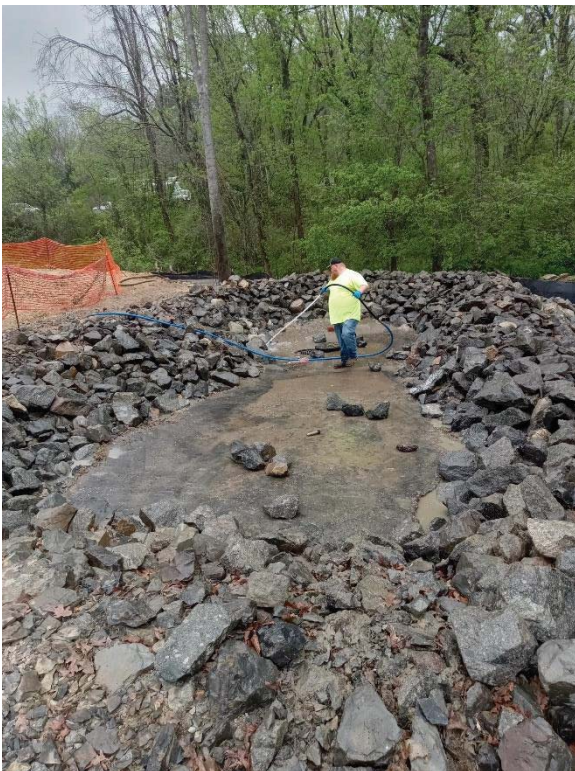
MH 1750 – Hydro-cleaning containment berm
