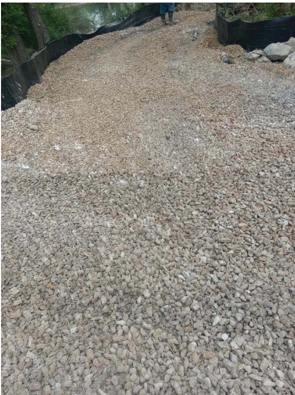
MH 1750 – Access road after cleanup
