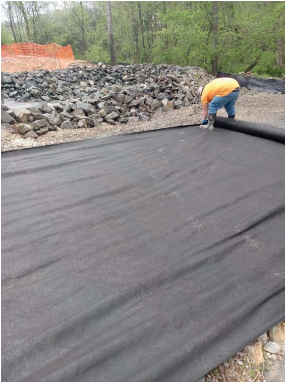
MH 1750 – Installing new liner in berm area
