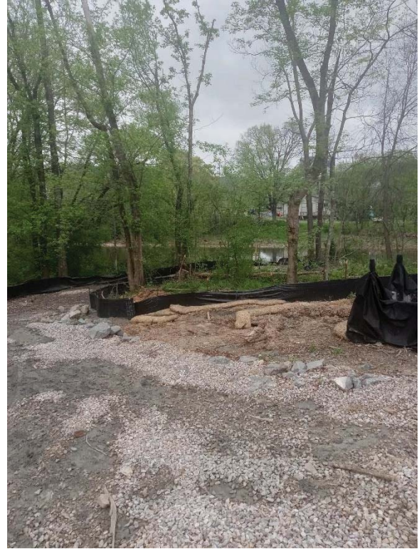
MH 1750 – Access before cleanup
