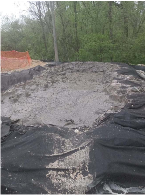
MH 1750 – Sludge inside berm after SSO stopped
