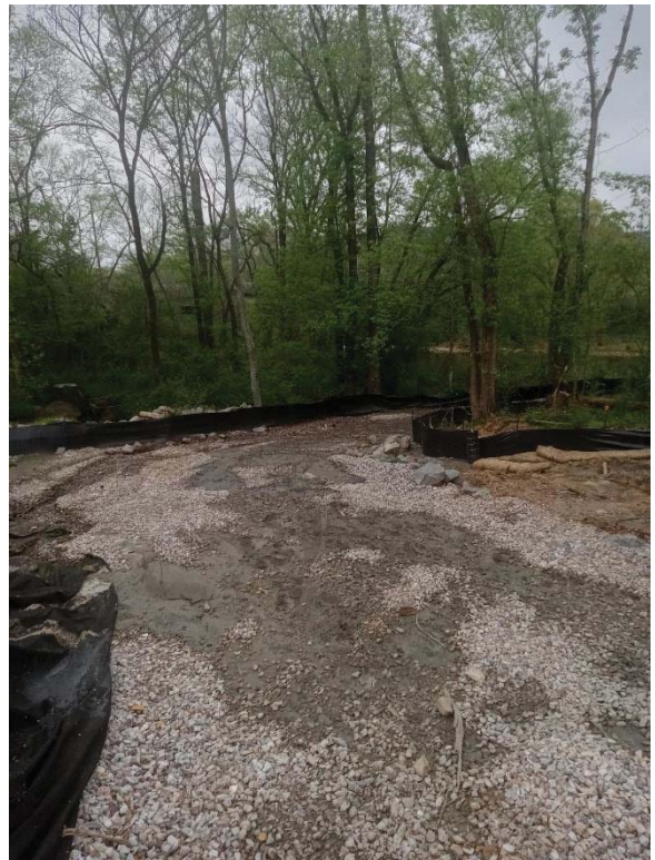
MH 1750 – Access road before cleanup
