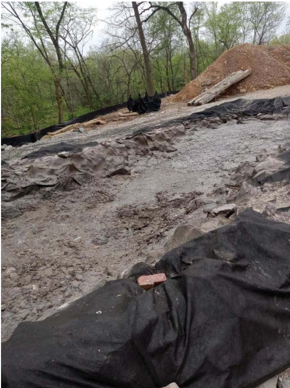
MH 1750 – Inside berm before cleanup
